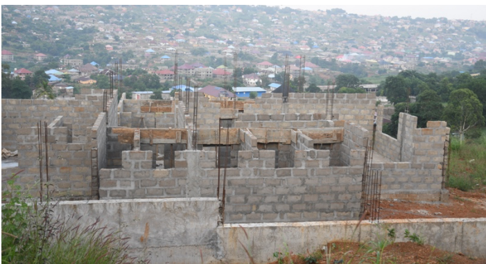
Figure 2: Ongoing construction of the Rainbo Centre of Excellence
